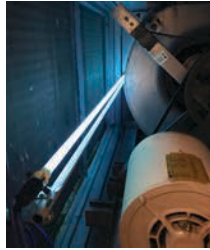
UV-C light keeps coils free of mold
